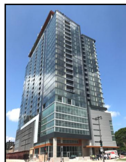
2022 Ascent skyscraper in Milwaukee certified as the world's tallest timber building at 25 stories, 86.6 metres (284 feet)
